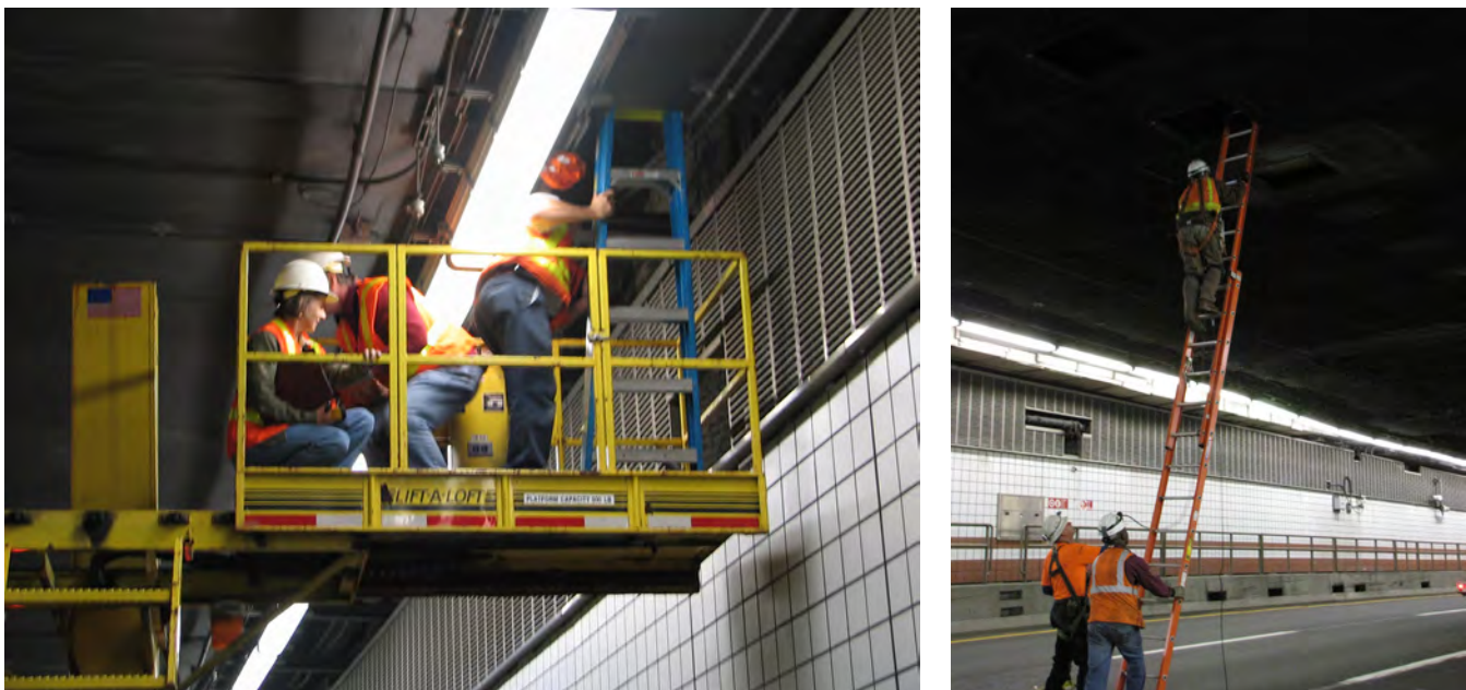
Figure 2.5 Equipment and location of access for tunnel inspection
