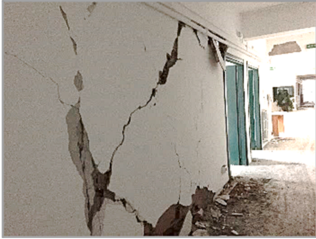
Fig. 16. Image of Lo2-type partition panel situated in the C/6-C/7 span on ground storey taken after 30th October 2016 earthquake.
