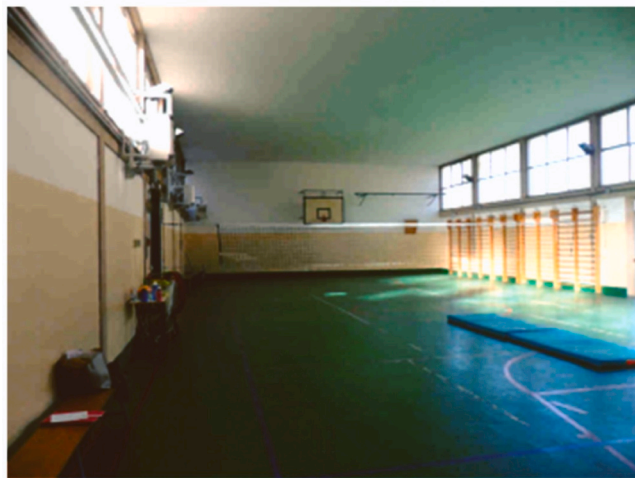
Fig. 1. External and internal views of case study building.
