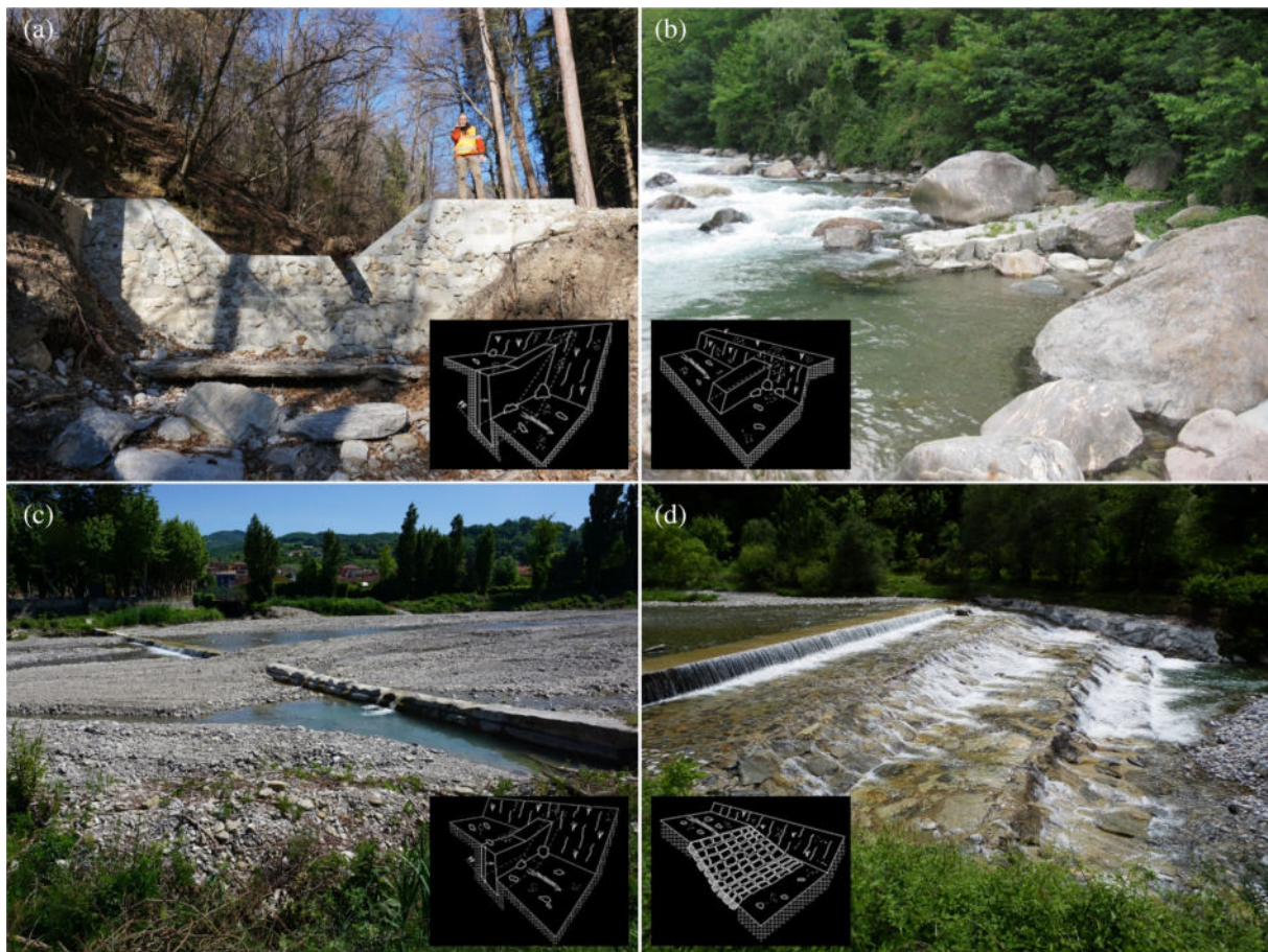
FIGURE 2 Photographs and illustration of transverse torrent control structure types: (a) check dam, (b) groyne, (c) sill, and (iv) bed protection structures (modified from Paratscha et al., 2019).
