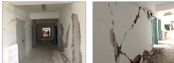
Figure 11. Images of the ground storey Lo2-type longitudinal partitions taken after 30 October 2016 earthquake
