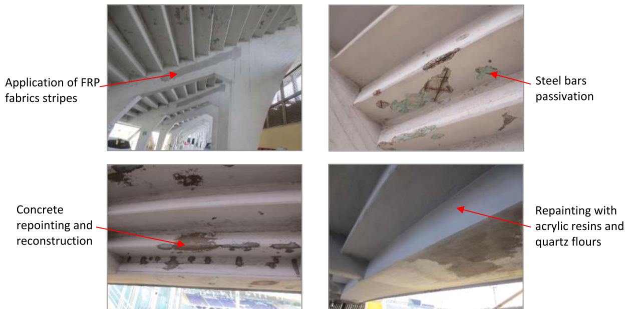
Fig. 17. Local static strengthening and restoration interventions.
