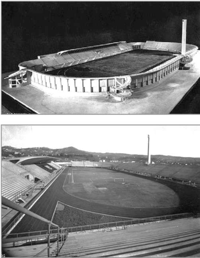
Fig. 1. Final architectural model of the Stadium, and internal view in 1932 (photographic archive Barsotti, Florence).
