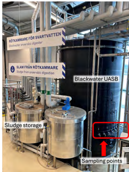
Figure 1. Pilot-scale UASB treating Blackwater at RecoLab, Helsingborg.
