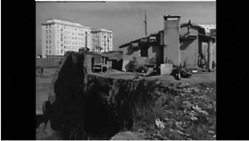
Figure 8.3. Mediating townscape and countryside. Ai margini della città (On the edge of the city, dir. Giorgio Ferroni, IT, 1954).
