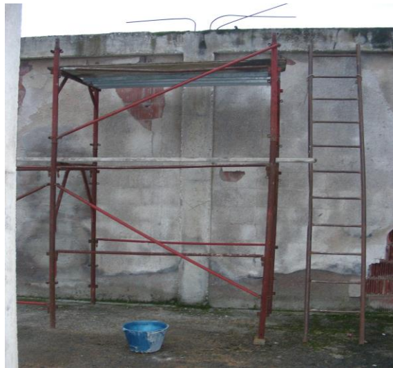
Photo 1 – Work place and scaffold
