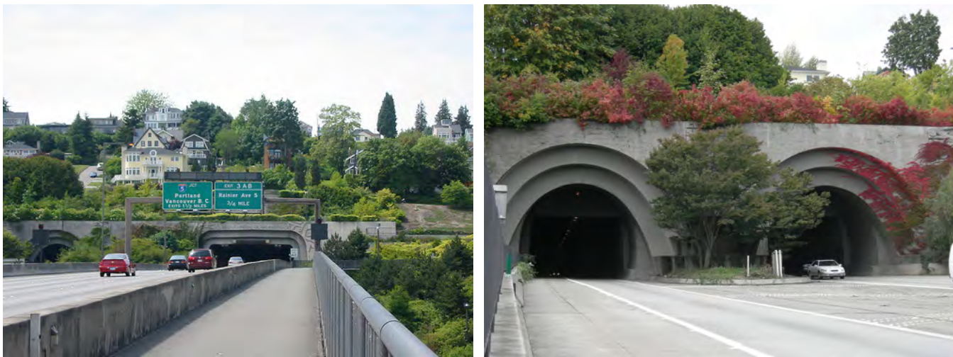
Figure 1.5 Mount Baker Ridge Tunnel on I-90 in Seattle
