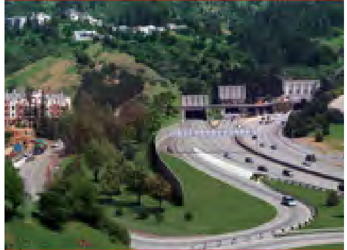
Figure 1.1 Fourth two-lane Caldecott Tunnel bore on SR-24 under construction
