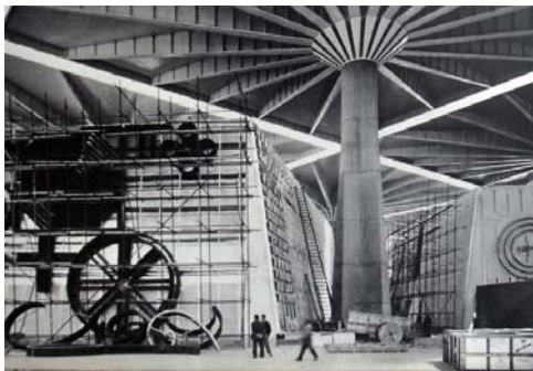
3. Nervi's structure internal view. In the centre of picture there is the wall set up by Fausto Melotti, from «Domus», no.380, July, 1961.
