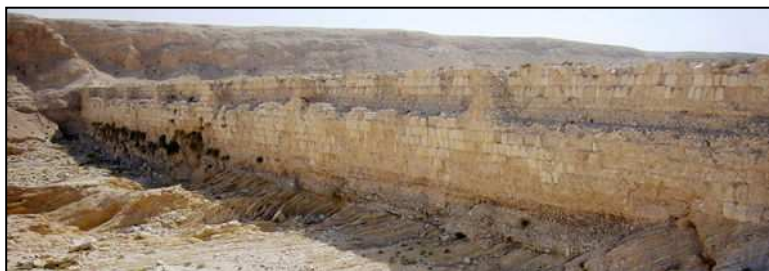
Fig. 4.5. A typical gravity dam: Harbaqa's one
