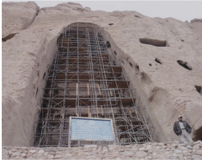
Fig. 4.51. Bamiyan Valley (Afghanistan), the reinforcement of one of the niches, after the dynamites
