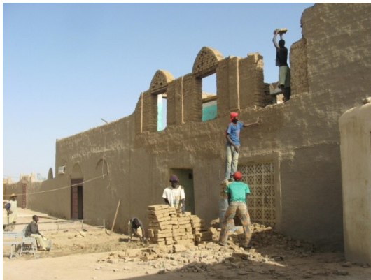
Fig. 4.28. Djenné (Mali), the reconstruction of the South façade
