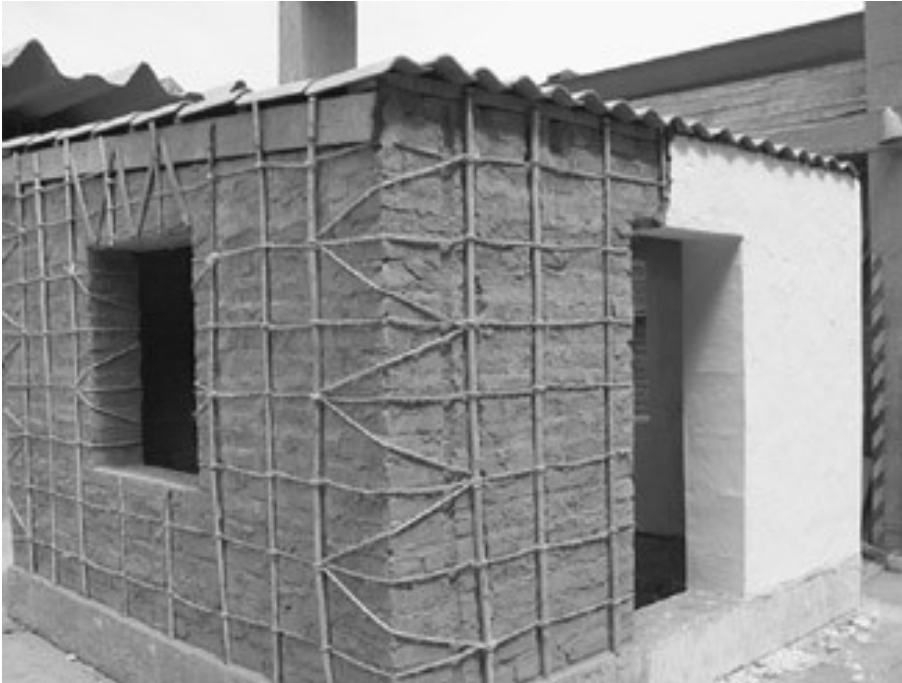
Fig. 5.60. Peru, implementation of natural mesh made by bamboo and rods
