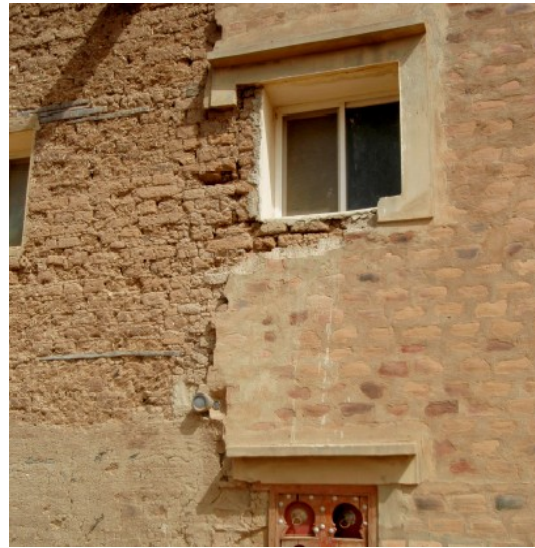
Fig. 4.41. Djenné (Mali), the damages of an earthen masonry, plastered with terracotta bricks
