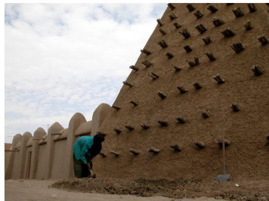
Fig. 4.22. Djingerey-ber (Mali), the conservation activities of the mosque
