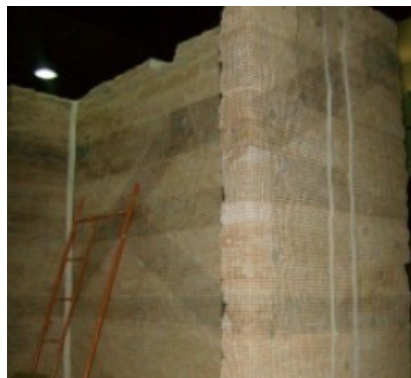
Fig. 5.62. Reinforcement of adobe wall with a synthetic mesh
