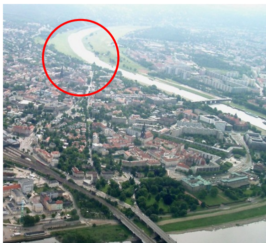
Fig. 3.14. The area chosen for the construction of the bridge
