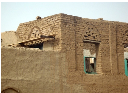
Fig. 4.30. Djenné (Mali), the original openings were restored
