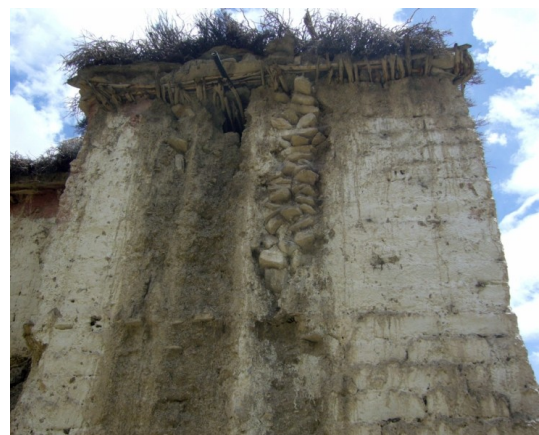
Fig. 5.3. Kanji, Ladakh (North India), wall erosion due to the water from the slope
