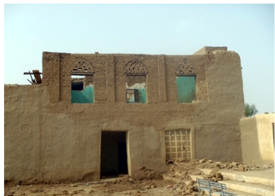
Fig. 4.31. Djenné (Mali), the original openings were restored
