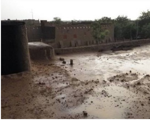
Fig. 5.10. Djenné (Mali) the Youth House: the water stagnation on the roof
