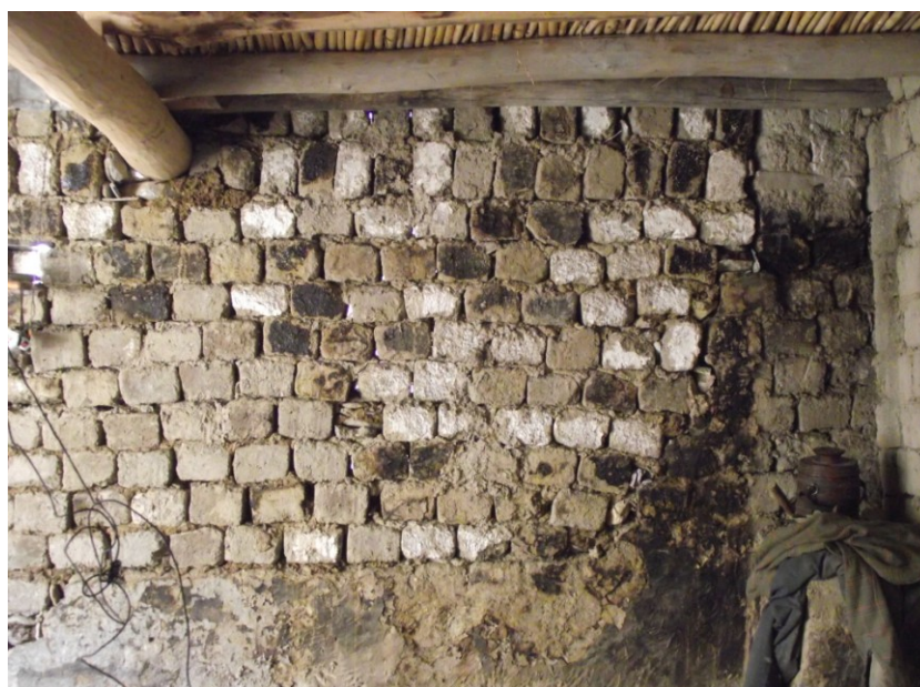
Fig. 5.52. Kanji (North of India), a house wall totally dismantled and rebuilt
