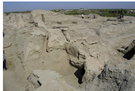
Fig. 5.9. Uch Kulakh (Uzbekistan), South-East bastion of the earthen castle in 2008
