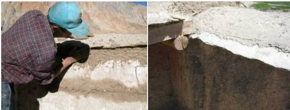
Fig.8-9. Creation of the protective stone cap and upper part in earth along the external edges of the perimeter wall.
