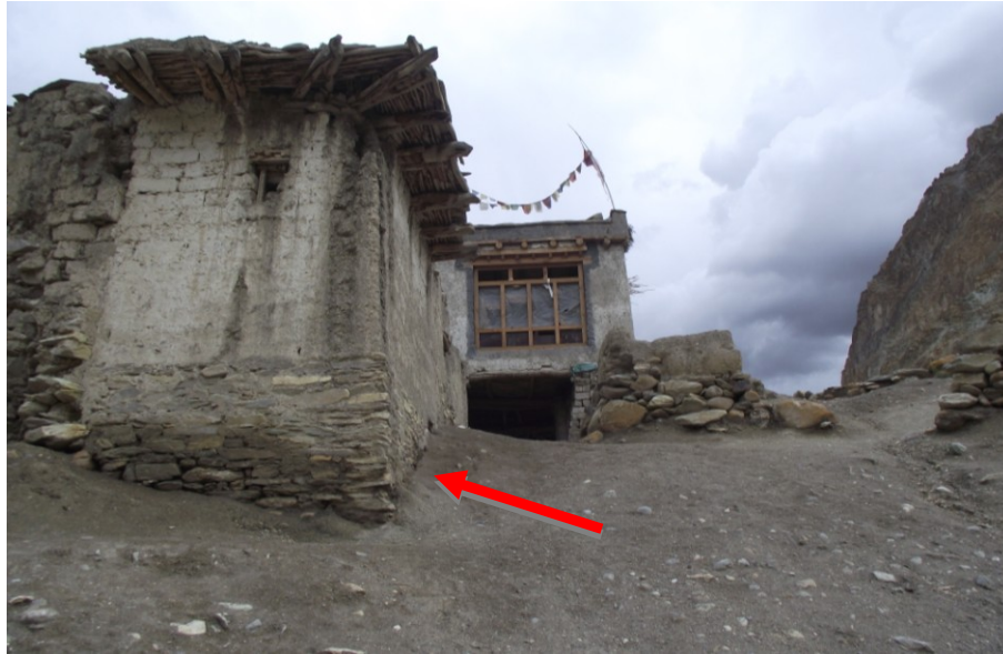
Fig. 5.39. Kanji, Ladakh (North India), the earthen buildings in this area are characterized by a stone basement without foundations
