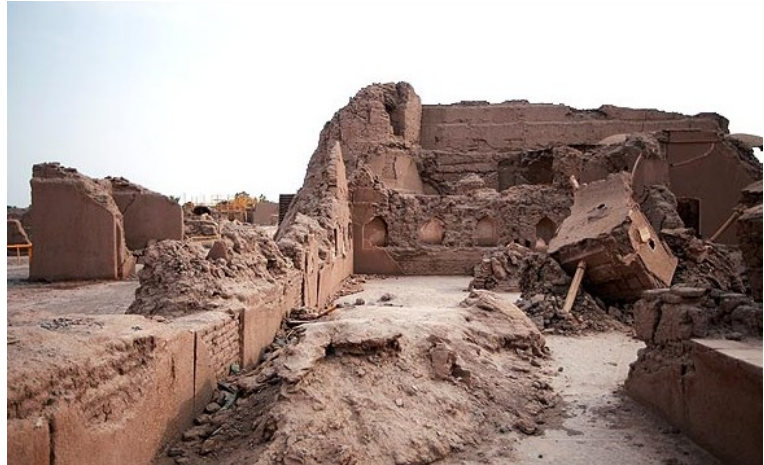
Fig. 4.57. Bam (Iran), after the 2003 earthquake
