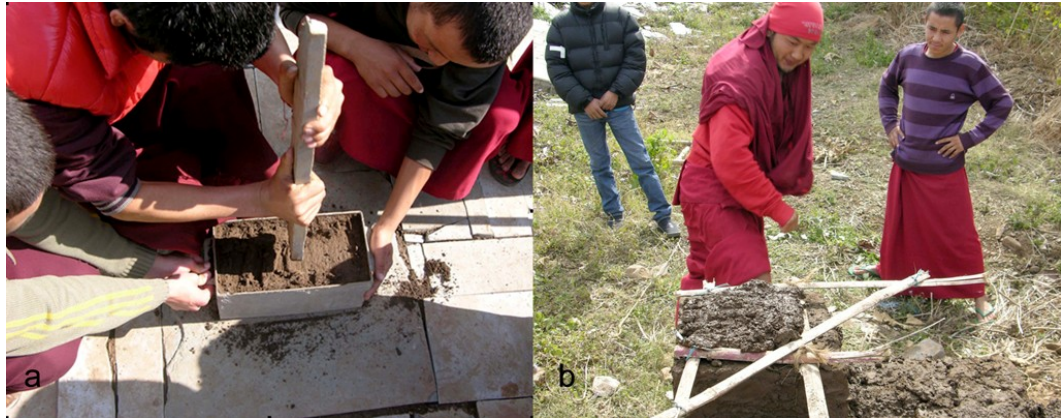
Fig. 6. Dehradun, India, the winter workshop: (a) the production of different pakbu and; (b) the improved corner joint of the walls due to a simple structure constituted by a band with two timbers in parallel and diagonal members for bracing at corners (credits: Mauro Bertagnin, 2011)
