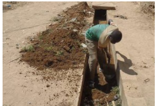
Fig. 4.17. Djenné (Mali), the clearing of the surrounding canals
