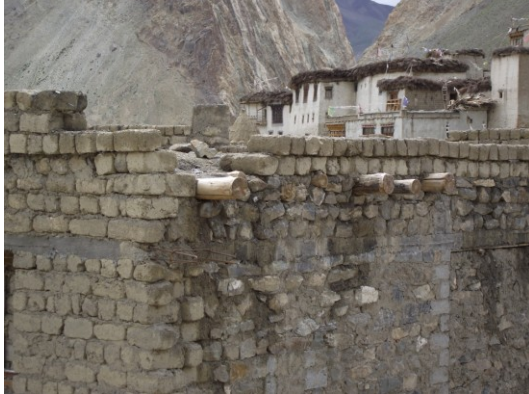
Fig. 4.45. Kanji (North India), a concrete curb in an earthen house
