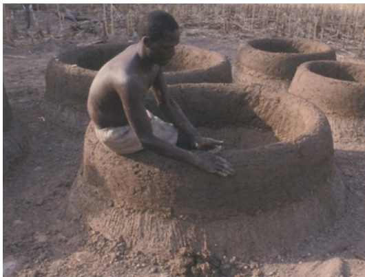
Fig. 4.10. Koutammakou (Togo), the implementation of the cob technique
