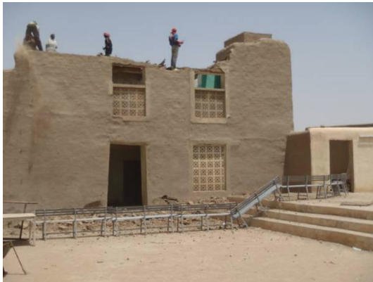
Fig. 4.26. Djenné (Mali), the dismantling of the South façade (starting phase)
