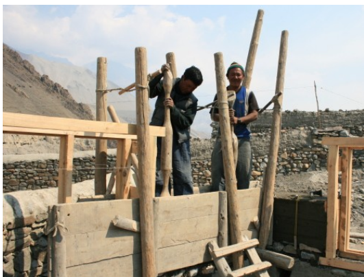
Fig. 4.4. Kagbeni (Nepal), the manual implementation of the rammed earth technique
