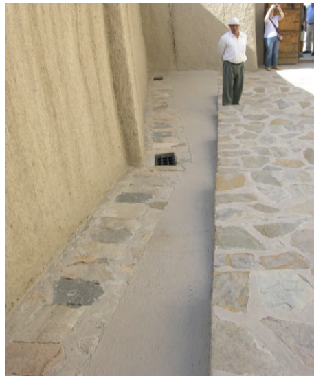
Fig. 5.36. Bahla fort (Oman) two different solutions of drainage with stones at the wall base and with stone and cement pavement
