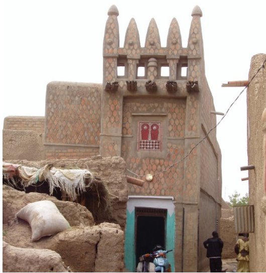
Fig. 4.40. Djenné (Mali), an earthen building totally covered with terracotta bricks
