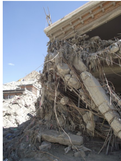
Fig. 5.4. Leh (North India), the disaster after the flood in 2010
