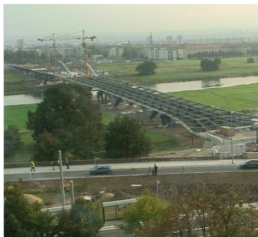
Fig. 3.15. The bridge construction works in September 2011
