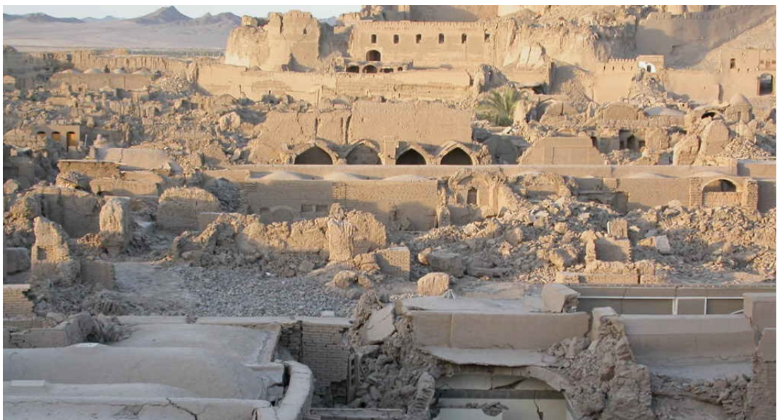
Fig. 4.58. Bam (Iran), after the 2003 earthquake
