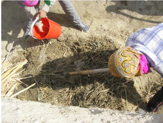
Fig. 5.56. Uch Kulakh (Uzbekistan), the preparation of the mixture: loam and dry palustrine cane
