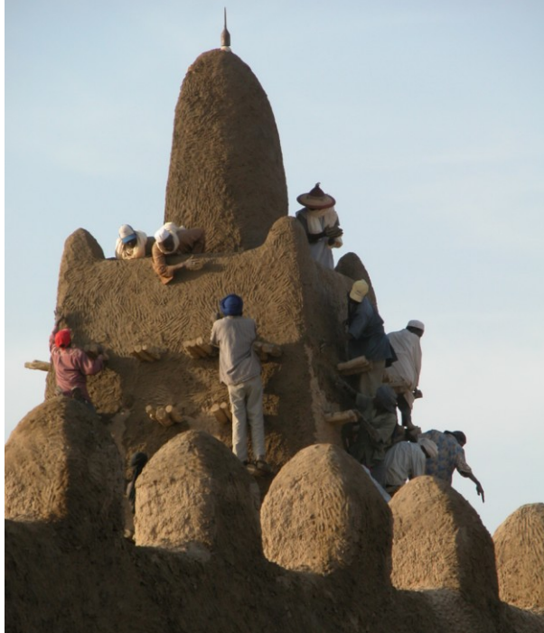
Fig. 5.73. Timbuktu (Mali), the periodical plastering of the mosque
