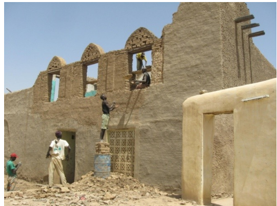
Fig. 4.29. Djenné (Mali), the reconstruction of the South façade
