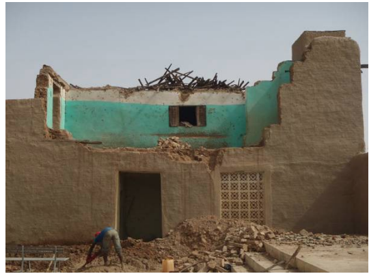
Fig. 4.27. Djenné (Mali), the dismantling of the South façade (ending phase)
