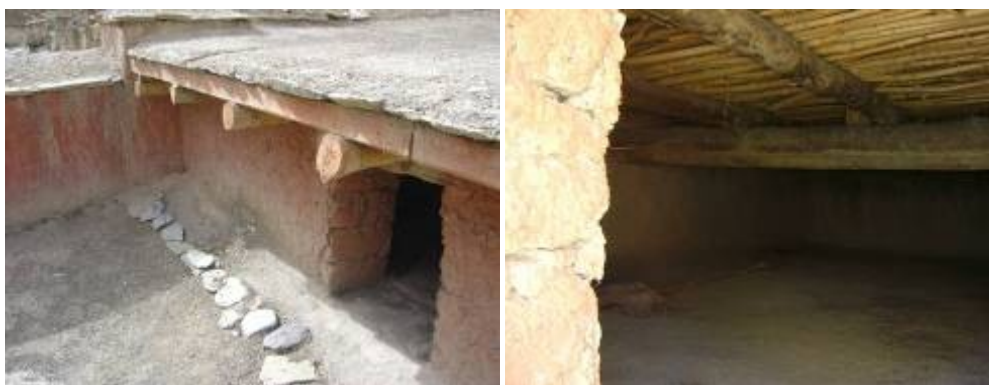
Fig.12-13. Intervention of the realised counter roof
