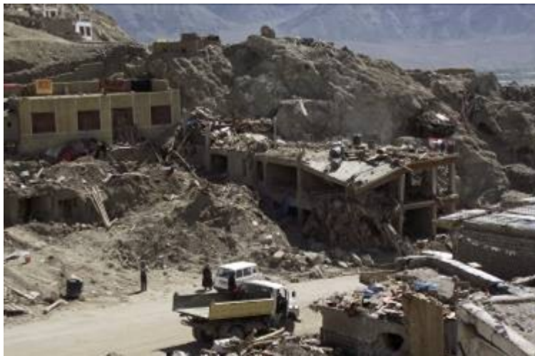
Fig. 1. Leh, Ladakh: the destruction of the urban fabric after the heavy monsoon and related flood (credits: Désirée De Antoni, 2010)
