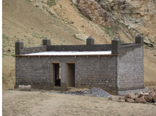
Fig. 4.46. Kanji (North India), the new women meeting point, built with stones and cement instead that with adobe, wood and stone
