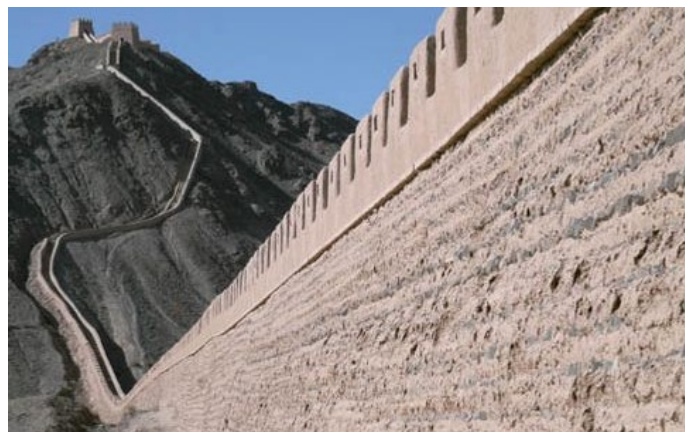
Fig. 4.53. The Great Wall in China, adobe and rammed earth sections
