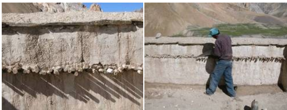
Fig.4-5. Cutting the protruding wooden elements along the perimeter wall.
