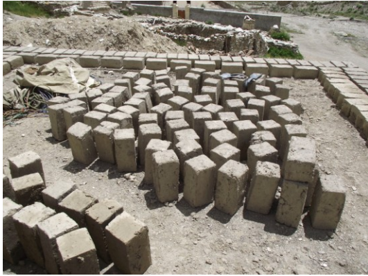
Fig. 4.2. Kanji, Ladakh (North India), the drying of the adobe
