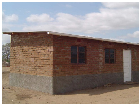
Fig. 4.13. Maputo (Mozambique), rural house made of CEBs
