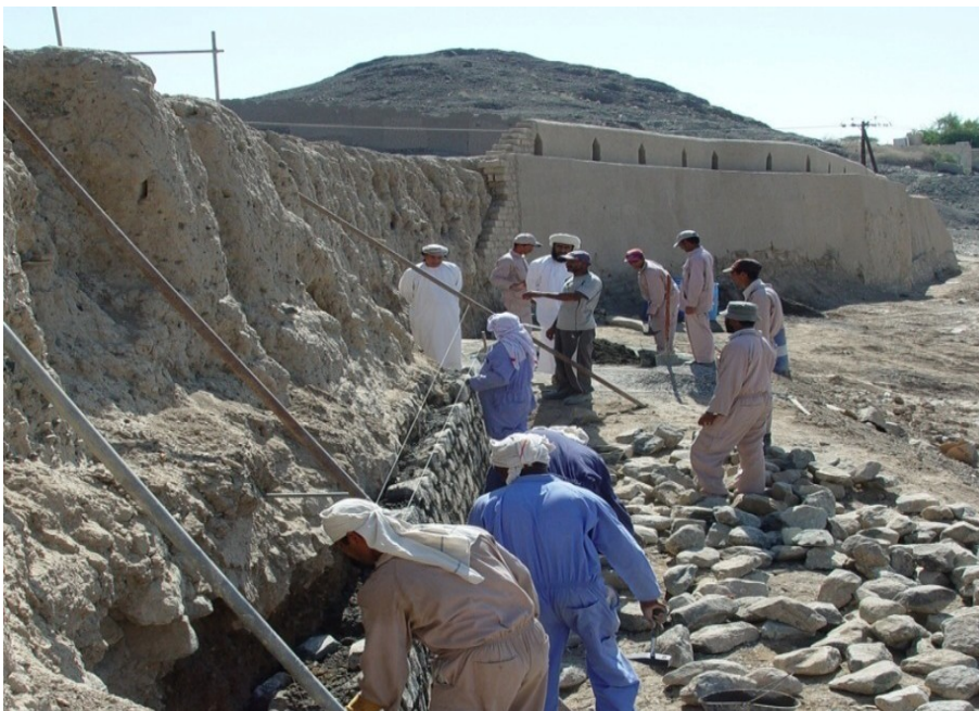
Fig. 5.38. Bahla (Oman), realizing a stone basement to stabilize the wall
