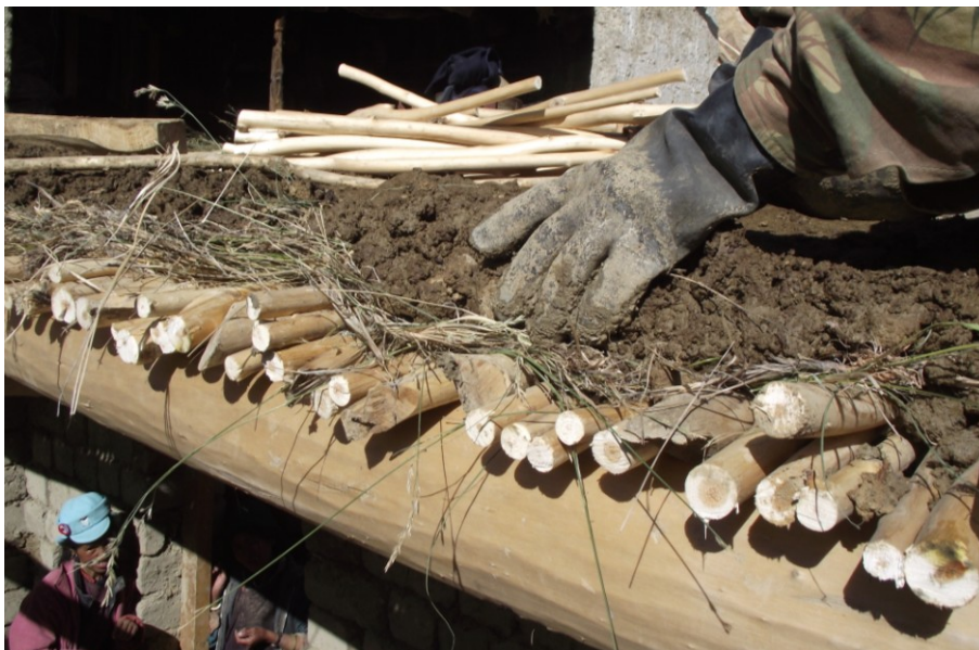
Fig. 5.86. Kanji, Ladakh (North India), the implementation of the roof
