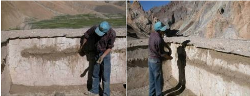
Fig.6-7. Plastering and correction along the line.
