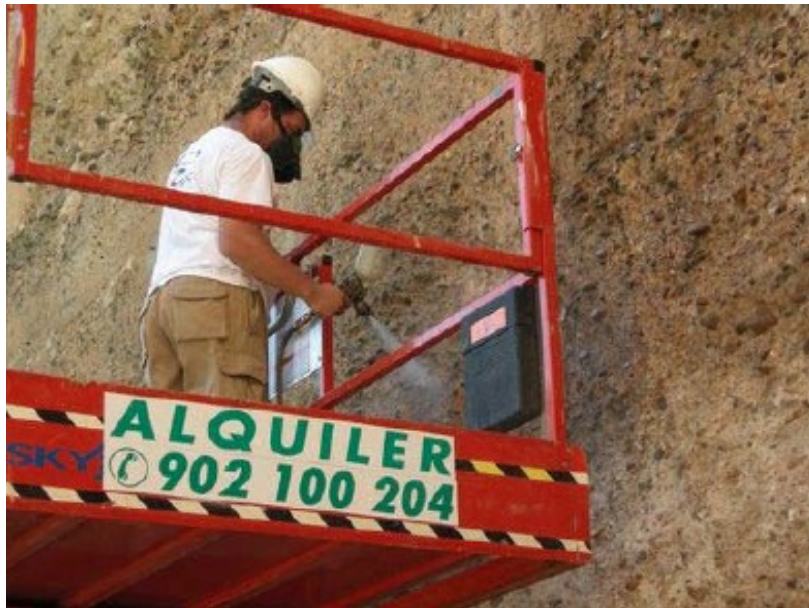
Fig. 5.77. Seville (Spain), ethyl silicate injection through an aerosol gun on a rammed earth ( tapial ) wall
