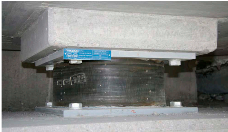
Fig. 2.33 – High damping Rubber Bearing (HDRB), 1991, archivio prof. James M. Kelly.
