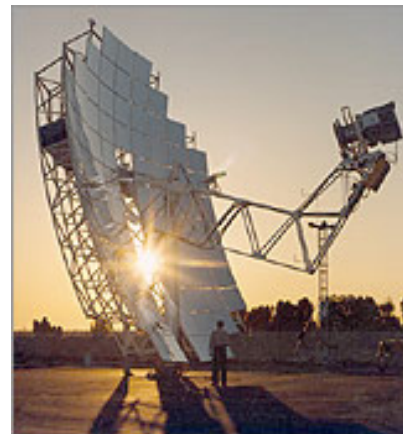
Figure 3.11: Left: Solar dish concentrator. Right: Solar dish system.
