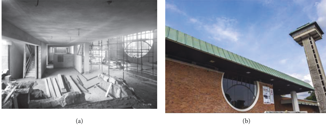
FIGURE 3: Glass facade (a) at the time of building construction (indoor view) and (b) today (outdoor view).
