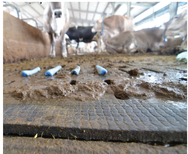
Fig. 5. Detail of the rubber liner used on top of the slatted floor in some areas
